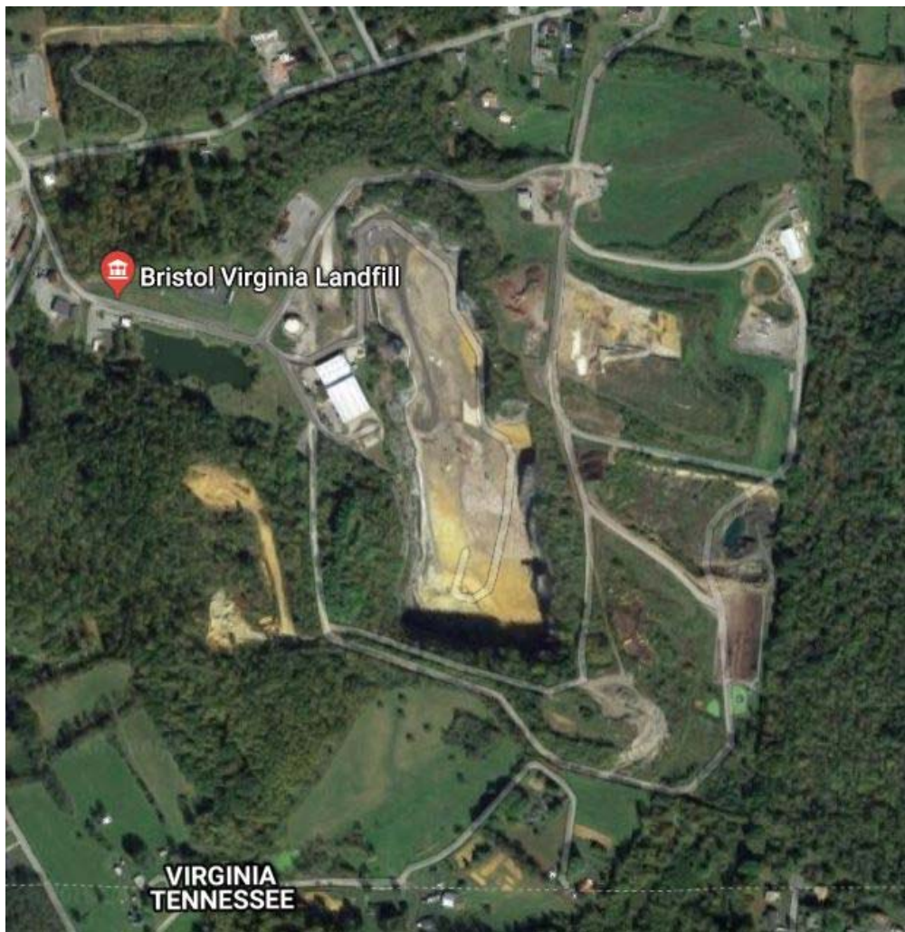
Exhibit 1. Bristol Integrated Solid Waste Management Facility (ISWMF)
